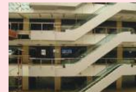
Cladding For Staircase Wall
